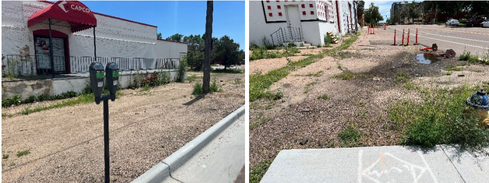
Figure 13. Lack of Sidewalks and Curb
