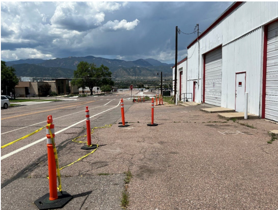
Figure 5. Excessive Curb Cuts Along Commercial Blocks
